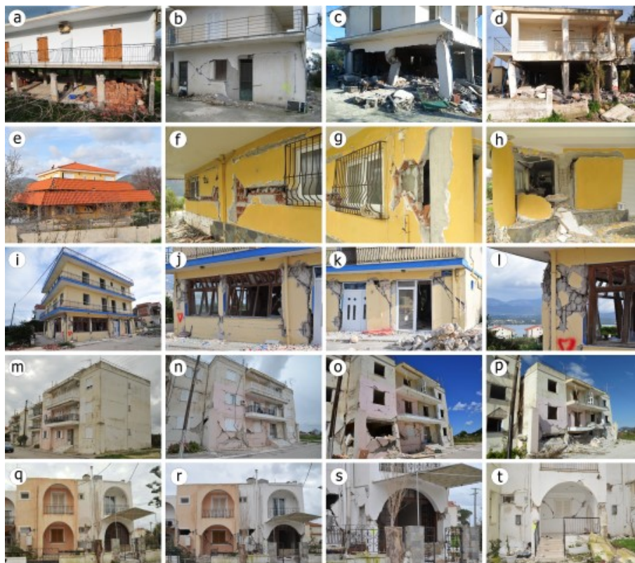
Fig. 6 – Damage to RC buildings. (a) A two-storey RC building in the Agios Dimitrios village suffered soft-storey failure on the verge of collapse, while the second storey remained intact. (b – d) A two-storey RC building in the Agios Dimitrios village suffered diagonal cracks and detachment of infill walls of the first floor from the surrounding RC frame by the first earthquake (b) and failure of columns and joints by the second earthquake (c, d). (e – h) A three-storey building sustained total collapse of the second floor due to absence of columns (e) and detachment of the infill walls from the surrounding RC frame due to vertically perforated bricks in the infill walls of the first floor (f, g, h). (i – l) A three-storey building in Lixouri probably built before 1984 sustained soft-storey failure, while the two upper floors remained also intact. (m – p) A three-storey building in the Lixouri public housing complex. The first earthquake caused moderate damage (m), while the second earthquake aggravated damage (n). (o, p) The same building on the verge of collapse in July 2015 and in November 2015
