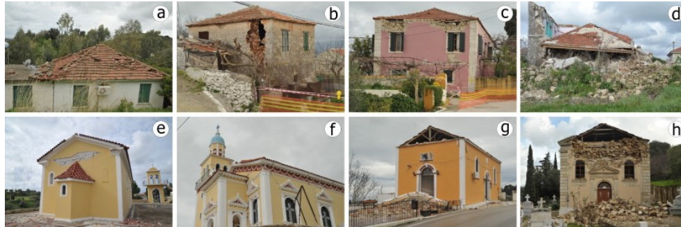
Fig. 7 – Damage to masonry buildings included (a) detachment of roof tiles, (b) partial collapse of the load bearing wall, (c) destruction of the upper corners of the buildings and (d) near total collapse of the building. Masonry churches suffered damage including (e) detachment of roof tiles and pieces of plaster, (f) cracks in masonry load bearing walls and in the upper corners of the structure and (g, h) fall of gables at the edge of double-pitched roofs.
