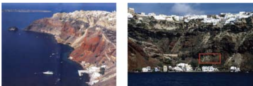
Figure 4. Views of Armeni bay. The dipping slopes with the morphological discontinuities, the impressive development of the scree fans and some minor extent intervention for landslides are notable. The settlement is characterized by high landslide risk that can be extended during seismic load.
