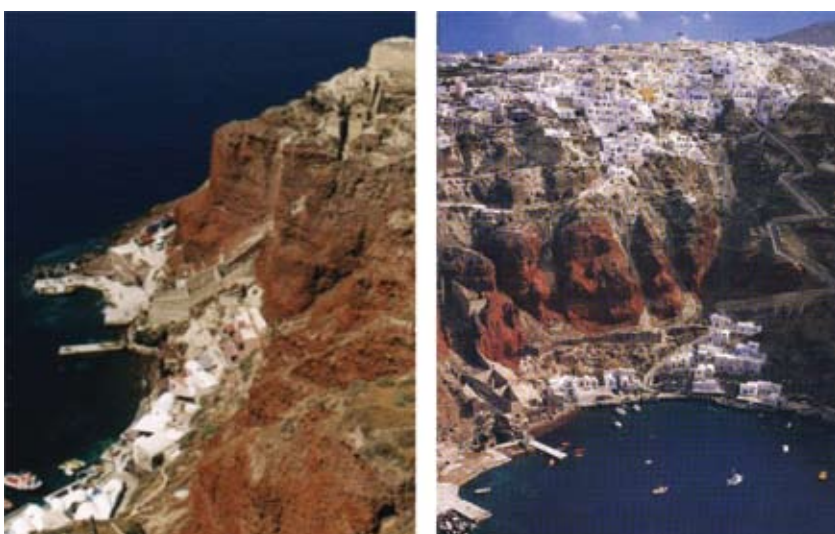
Figure 5. Views of the Ammoudi bay and the settlement of Oia. The steep slopes that the Scoriae formation forms can be viewed. In addition the supporting walls for the protection of the settlement from minor rockfalls and scree are showed. The settlement is in high risk due to the rockfalls and landslides that in case of an earthquake they can be extended.
