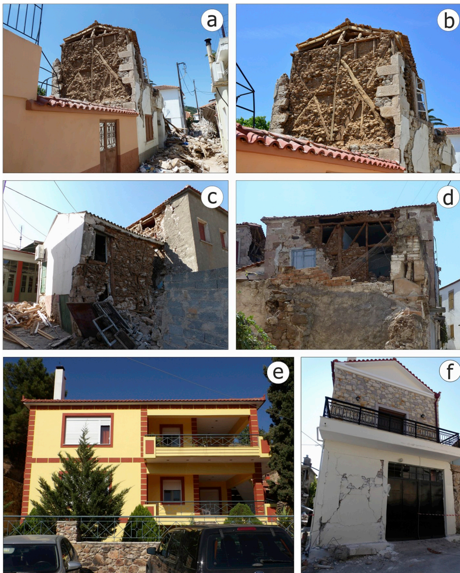
Fig. 11. (a–d) Traditional residential buildings with dual structural system including masonry walls and timber frames with extensive “X” bracing in Vrissa settlement (a–d). During an earthquake, these frames could guarantee the stability of the roof in case of a partial collapse of the masonry structure. This dual structural system represents one of the earliest surviving architectural responses to earthquake motion in Greece and Turkey and was also observed in Eressos and Bergama by Refs. [64,65]. (e–f) The R/C buildings showed good performance and remained almost intact (e) by the 2017 Lesvos earthquake. But there were exceptions (f) including cracks in the infill walls, detachment of large pieces of plaster from the infill walls of the ground floor as well as detachment of the infill wall from the surrounding RC frame.
