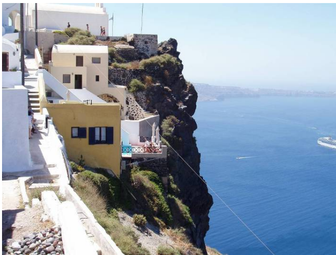
Figure 4. View of constructions founded on lava in the area of Skaros at the caldera brow in critical stability conditions.
