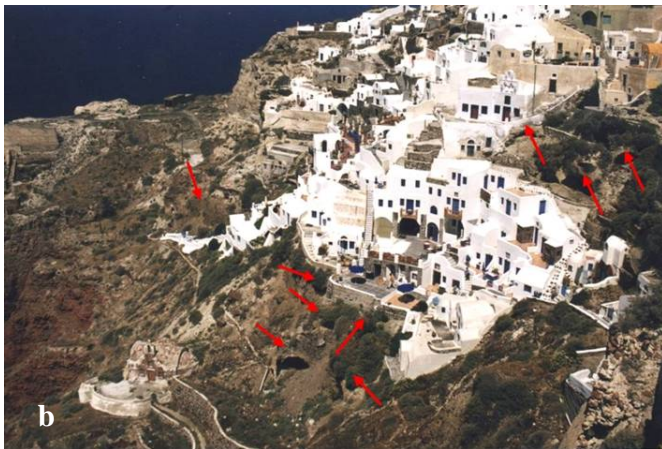
Figure 11. a. Views of Oia, town located over Ammoudi cove. b. Constructions on Upper Pumice slopes with high morphological dip values. The existing stability conditions are aggravated by the numerous caverns located under the constructions (arrows).
