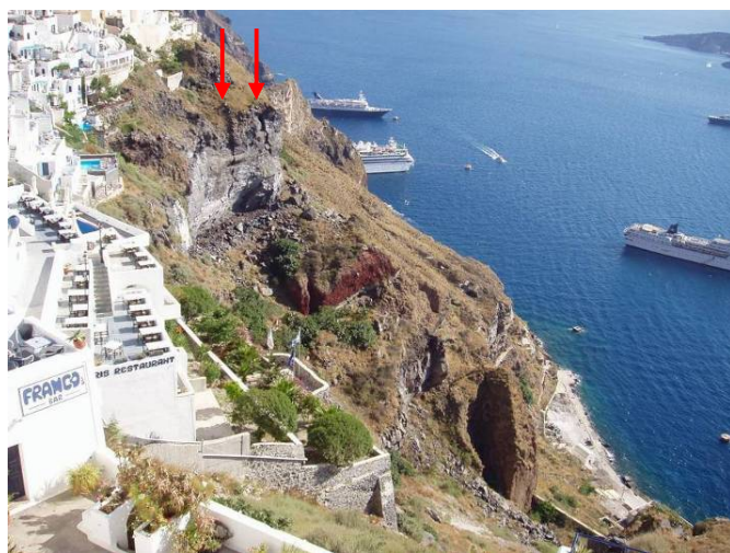
Figure 7. Views of the Pyroclastic Formations that compose the lower section of the slopes under Fira town. The discontinuities that develop in the overlying lava formations (arrows) that increase landslide hazard can be observed.
