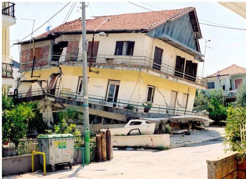
Fig. 15: A modern building toppled over. In the right hand side there are no brickwalls in the ground floor, where the building toppled. On the contrary the remaining part at the left hand side has partitions down to the foundation.
