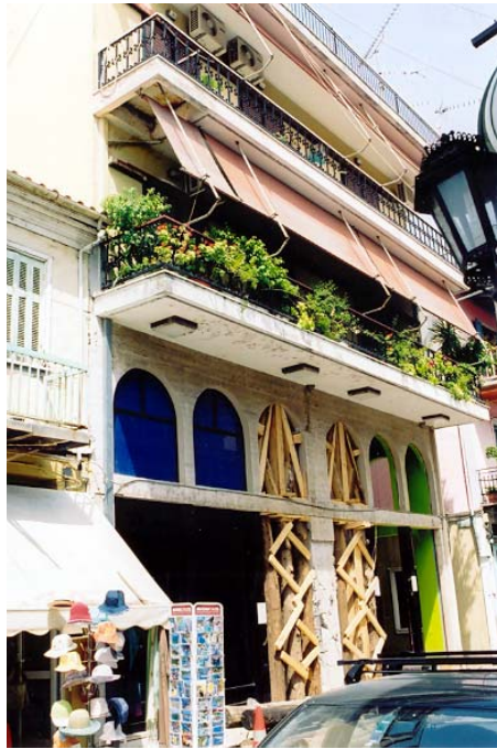
Fig. 19: A four storeyed building with a mezzanine was heavily damaged in the columns of the ground floor. The columns seem to have swollen in the centre due to insufficient transverse reinforcement.
