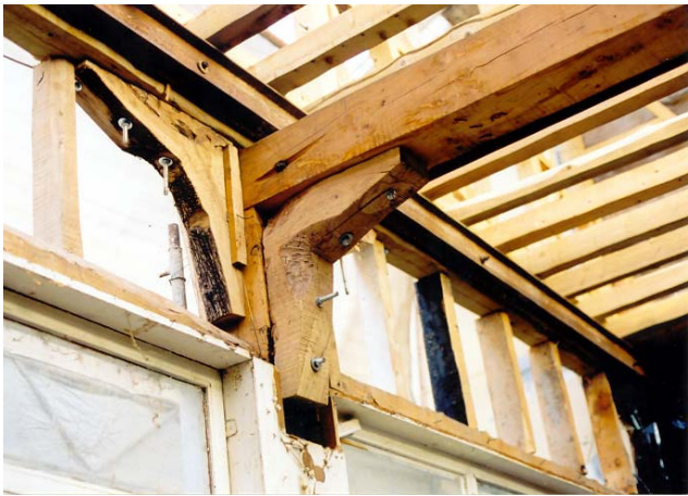
Fig. 14: The traditional earthquake resistant system of Lefkada. The building is at the end of the 19 th century. In Fig. 14b one may see the wooden columns and beams (w) with wooden corners (c). In Fig. 14c the special earthquake system under construction, is shown.
