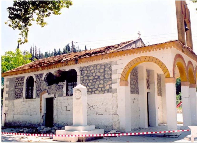
Fig. 16: Churches were build out of stone masonries. Suffered heavy damages. In various parts of Lefkada the roof tiles at the central part of the roofs were moved. This might be explained with the vertical flexibility of the roof at its centre.
