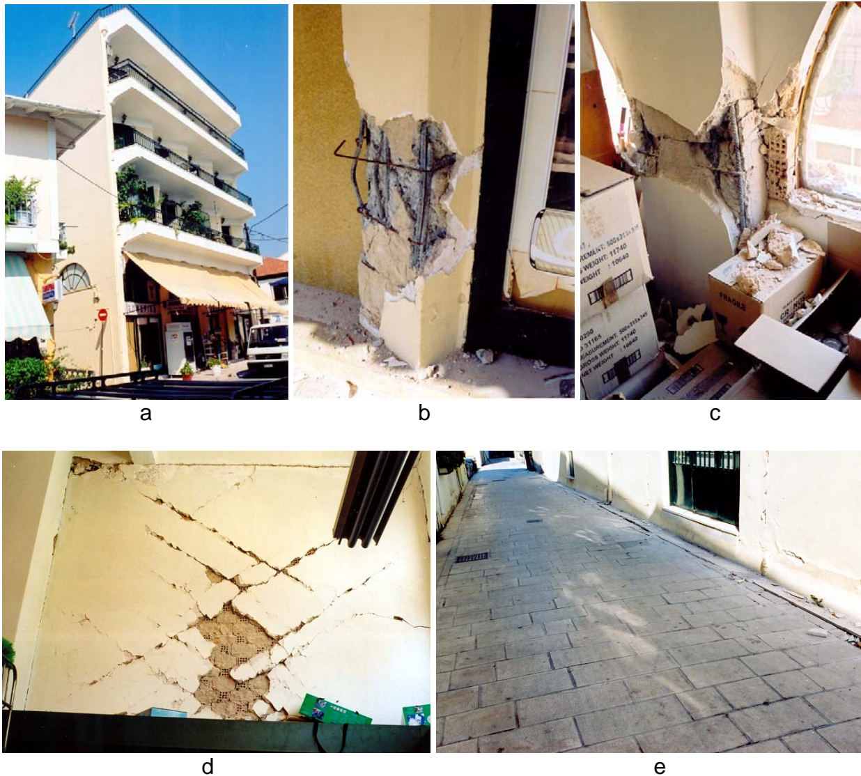
Fig. 18: A heavily damaged building in the city of Lefkada. The ground floor is a super market and has a mezzanine (a). The stirrups are insufficient and with wrong detailing (b). In the mezzanine the columns suffered also heavy damages on the surface between phases of concreting and in the lower part of the arches, formed with brickwalls (c). The inside brickwall partition in the ground floor absorbed a lot of energy and behaved as if it was reinforced (d). The building is on a pile foundation. A subsidence of few cm is shown in the figure (e).
