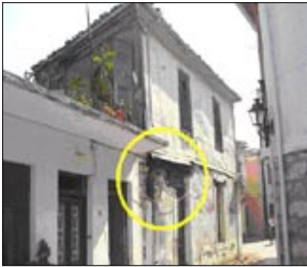
Figure 18. Partial collapse of masonry wall in a category B building (ITSAK team).
