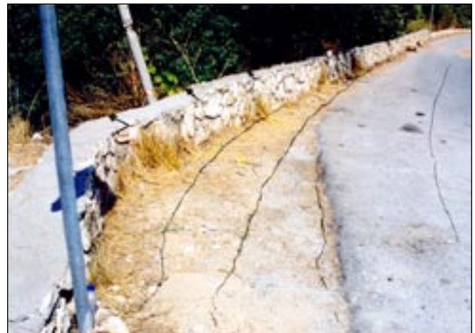
Figure 9. Many retaining walls leaned towards the external side; the adjacent parts of the roads subsided, and cracks appeared on the pavement (NTUA-UoA team).
