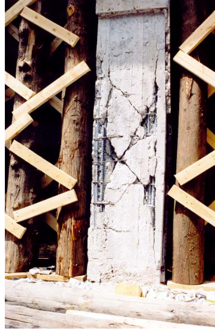
Fig. 19: A four storeyed building with a mezzanine was heavily damaged in the columns of the ground floor. The columns seem to have swollen in the centre due to insufficient transverse reinforcement.
