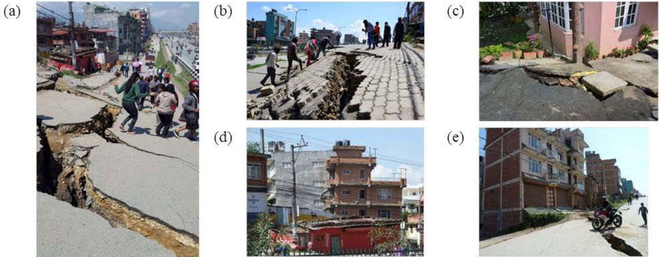
Fig. 2 – (a) View of a spectacular stretch of the central Nepal highly disrupted zone along the northern side of the Araniko Highway, Kathmandu city. The ground was deformed into a monocline escarpment with 1.6m of relief. Tension cracks were formed at the crest of the zone. (b) Another view of a monocline escarpment in area of tilted bricks along the northern pavement of the Araniko Highway. The ground on the right (NNW) lifted up about 1.3 m relative to the ground on the left (SSE). The crest of the escarpment was broken and discontinuous. Originally flat-lying pavement bricks and the cement slab were tilted near the crest of the escarpment. (c) The concrete yard was broken into polygonal pieces due to ground deformation, which were lifted upward due to N-S compression. Note that the house is unaffected. (d), (e) Many multi storied buildings were tilted without structural damage.
