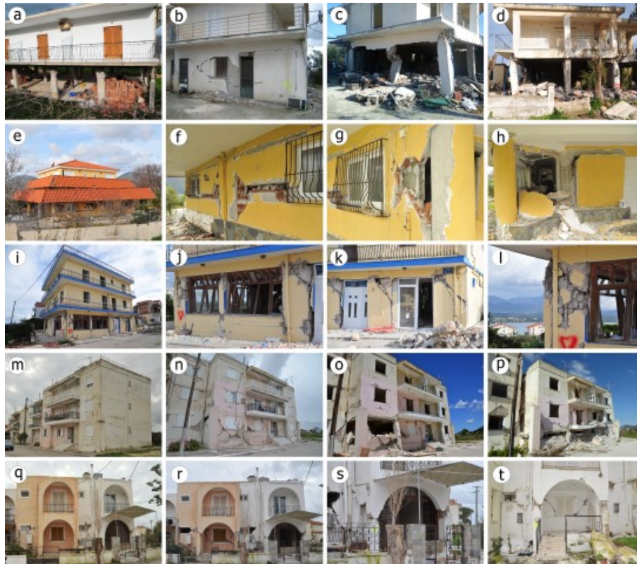
Fig. 6 – Damage to RC buildings. (a) A two-story RC building in the Agios Dimitrios village suffered soft-story failure on the verge of collapse, while the second story remained intact. (b – d) A two-story RC building in the Agios Dimitrios village suffered diagonal cracks and detachment of infill walls of the first floor from the surrounding RC frame by the first earthquake (b) and failure of columns and joints by the second earthquake (c, d). (e – h) A three-story building sustained total collapse of the second floor due to absence of columns (e) and detachment of the infill walls from the surrounding RC frame due to vertically perforated bricks in the infill walls of the first floor (f, g, h). (i – l) A three-storey building in Lixouri probably built before 1984 sustained soft-story failure, while the two upper floors remained also intact. (m – p) A three-story building in the Lixouri public housing complex. The first earthquake caused moderate damage (m), while the second earthquake aggravated damage (n). (o, p) The same building on the verge of collapse in July 2015 and in November 2015 immediately after the Mw 6.4 Lefkas (Ionian Sea, Western Greece) earthquake. (q – p) Another two-story building in the Lixouri public housing complex suffered moderate damage due to the first earthquake (q) and severed damage due to the second earthquake (r, s, t).
