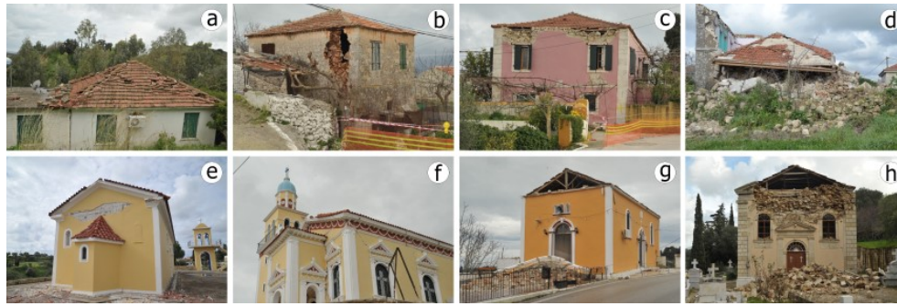
Fig. 7 – Damage to masonry buildings included (a) detachment of roof tiles, (b) partial collapse of the load bearing wall, (c) destruction of the upper corners of the buildings and (d) near total collapse of the building. Masonry churches suffered damage including (e) detachment of roof tiles and pieces of plaster, (f) cracks in masonry load bearing walls and in the upper corners of the structure and (g, h) fall of gables at the edge of double-pitched roofs.
