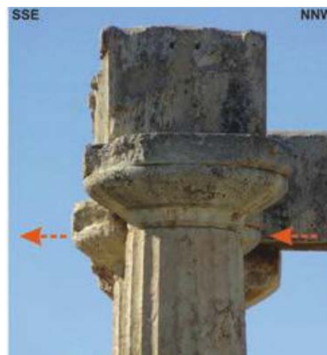
Figure 7: The capital of the column under the restored epistyle that preserves a displacement of ~ 10 cm towards the SSE.
