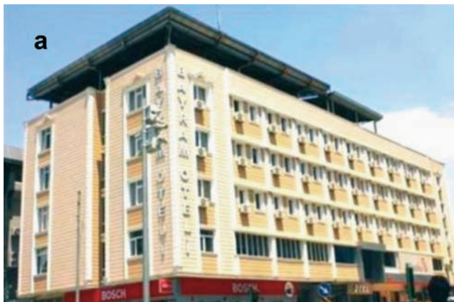
Fig. 30. a) The free standing Bayram Hotel before the earthquake and after the addition of a floor with a light weight roof. b) The collapsed roof is covering the plan, of the collapsed building in a parallel way to the pavements.
