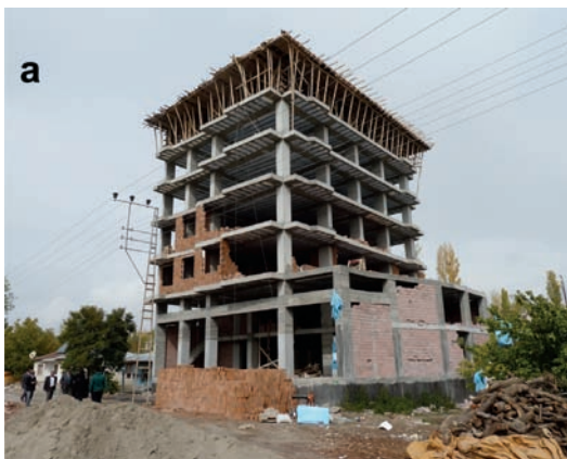
Fig. 19a, b. Flexible buildings with rather large openings and without shear walls, as well as those with a one way flat-slab construction system are prevalent in new structures.
