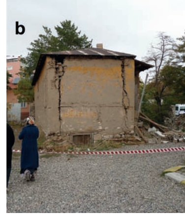
Fig. 16a, b. This manner of damage of simple houses indicates the dominance of vertical seismic component.
