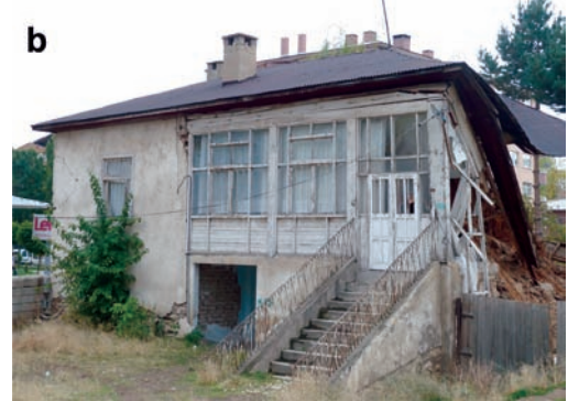
Fig. 16a, b. This manner of damage of simple houses indicates the dominance of vertical seismic component.
