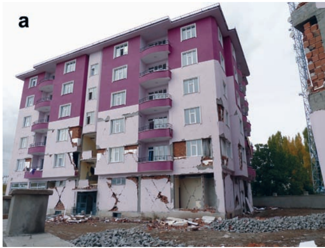
Fig. 28a, b. Note that the glass panels are intact while the walls are damaged especially at the lower levels. This is the case for almost the majority of the damaged-not collapsed multi-storeyed buildings, in Ercis city.
