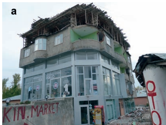
Fig. 20a, b. Usually, one or two storeys are added at the top and the balconies are externally closed with masonry partitions.
