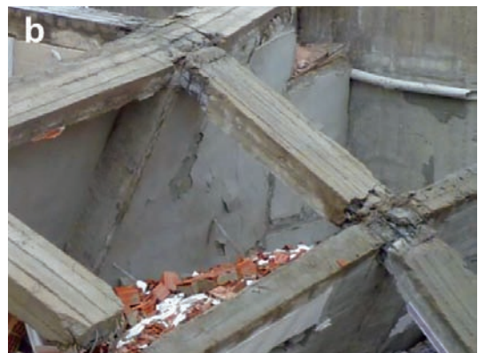
Fig. 25a, b. A technically interesting collapse. The reinforcement detailing is acceptable. Perhaps the concrete quality might have a problem or the concreting.
