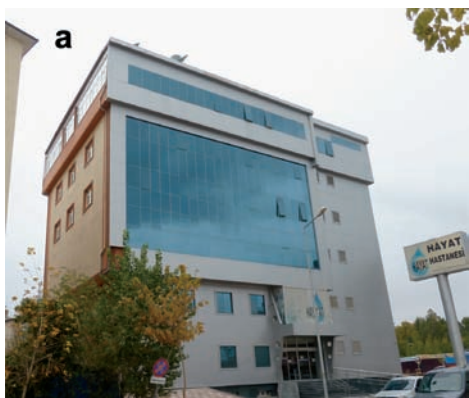
Fig. 22a, b. Externally, some well designed and constructed strong modern buildings, did not present any damage. Internally, the secondary elements and the content suffered extensive damage.
