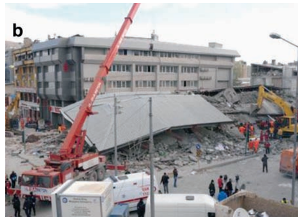
Fig. 30. a) The free standing Bayram Hotel before the earthquake and after the addition of a floor with a light weight roof. b) The collapsed roof is covering the plan, of the collapsed building in a parallel way to the pavements.
