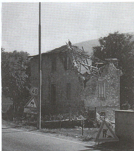
Figure 5. View of class B building and grade of damage 4, in the area of Casenova.
