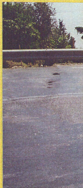
Fig. 14. The active fault of the southern margin of Tsambika beach. From the kinematic point of view this fault is characterized by creep movement and causes a lot of damages to the Rhodes - Lindos national road.
