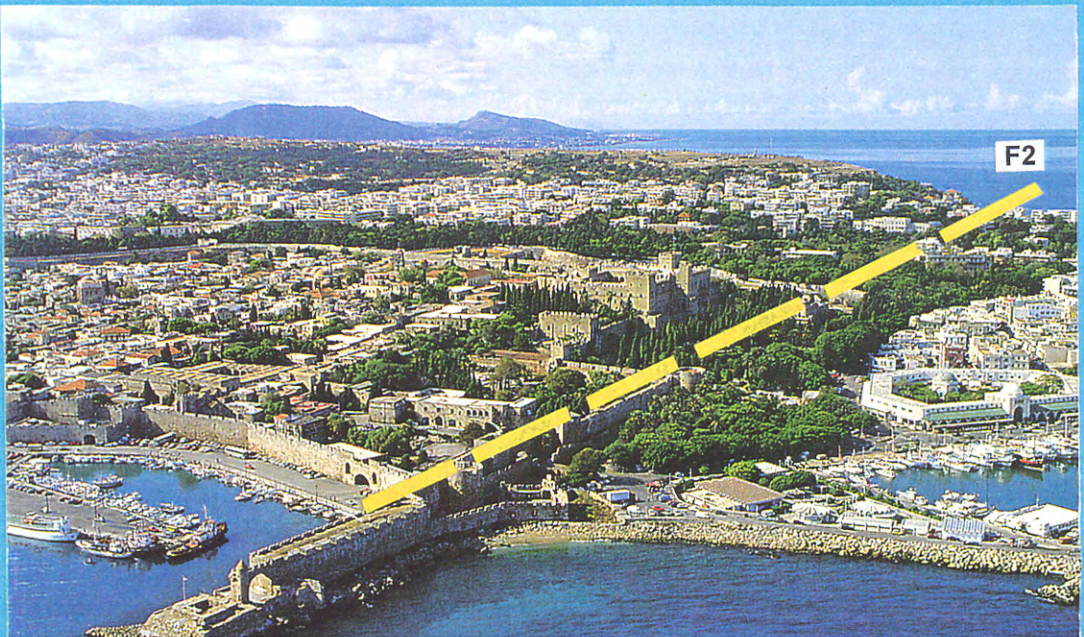
Fig. 5. View of the City of Rhodes with the Old Town and the M. Smith hill. The F2 fault zone is running along the northern slope of M. Smith, through the houses and the Medieval Trench.
