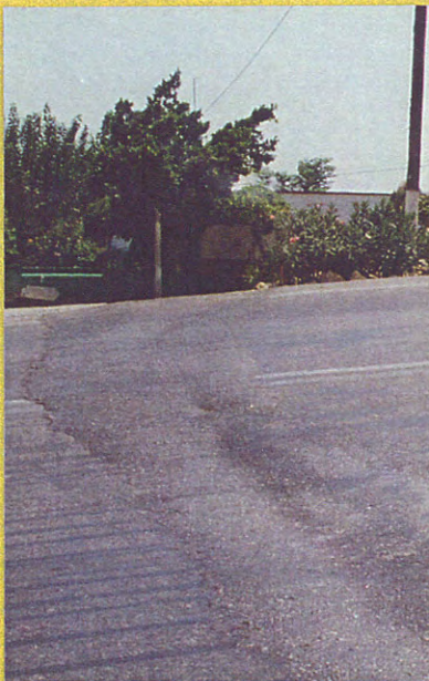
Fig. 14. The active fault of the southern margin of Tsambika beach. From the kinematic point of view this fault is characterized by creep movement and causes a lot of damages to the Rhodes - Lindos national road.
