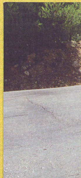
Fig. 14. The active fault of the southern margin of Tsambika beach. From the kinematic point of view this fault is characterized by creep movement and causes a lot of damages to the Rhodes - Lindos national road.
