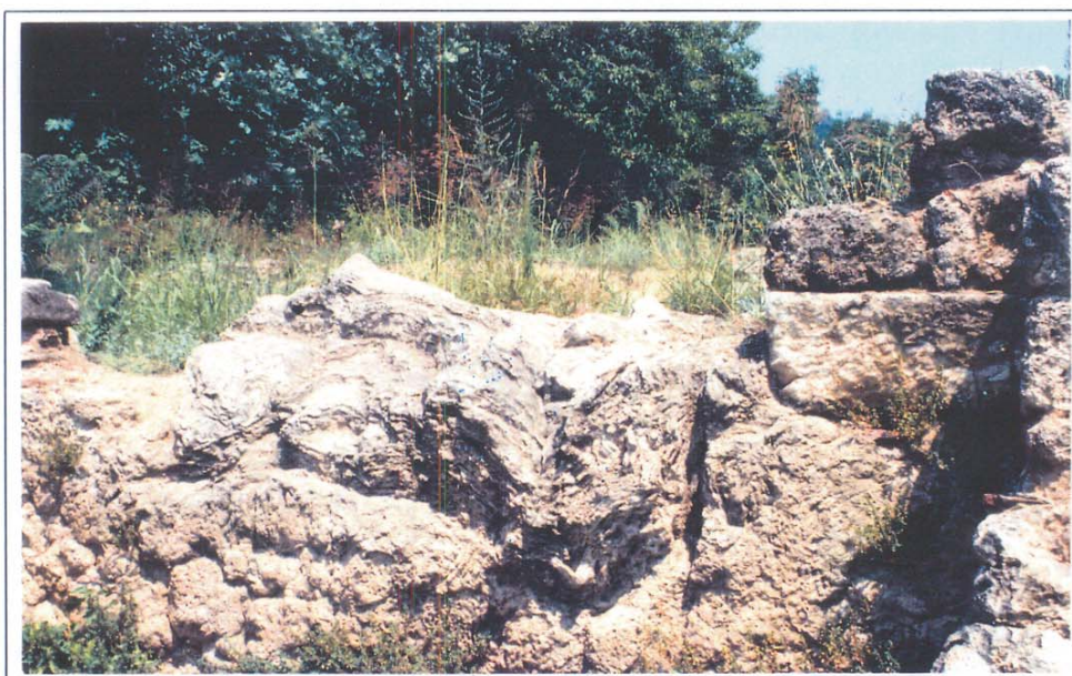
Figure 4. Travertine limestone with extraordinary erosional features of ‘V’ type on the flagstones of the fortification wall of the “Kato Polis”.
