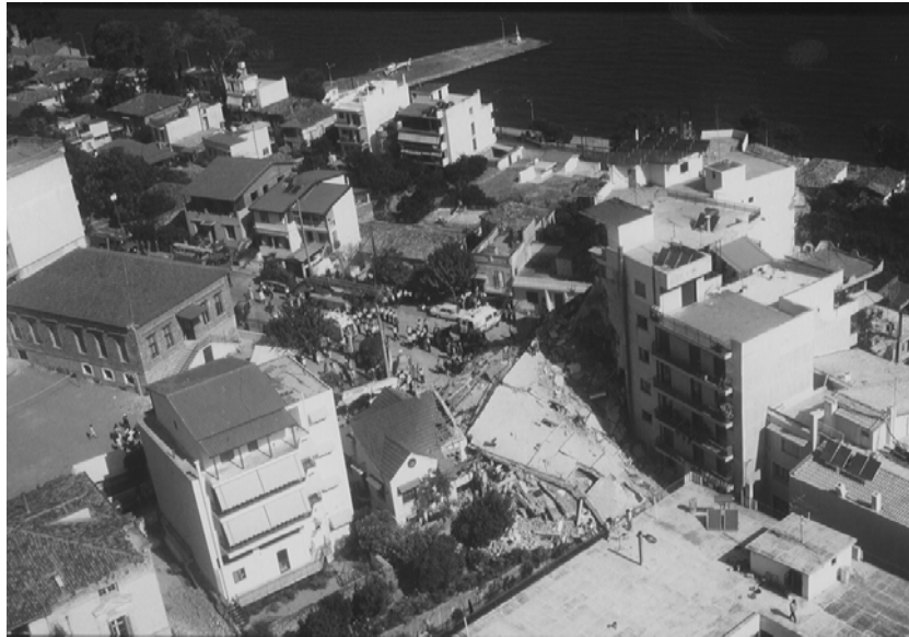
Figure 4. Aerial view of the collapsed apartment block. The port of Egio can be seen in the background. The Egio fault scarp runs from the top left to the middle right of the photo, directly beneath the row of buildings
