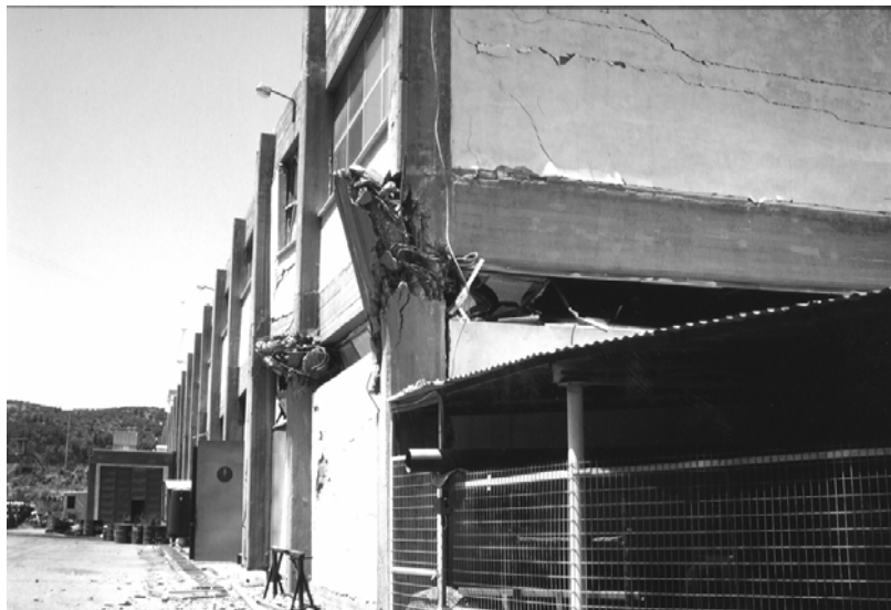
Figure 5. Severe structural damage at the building of Hellenic Weapon Industry.
