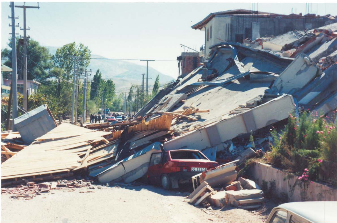
Fig. 4 Collapse of a multistorey R/C building at central Dinar where thin, loose formations are present.
