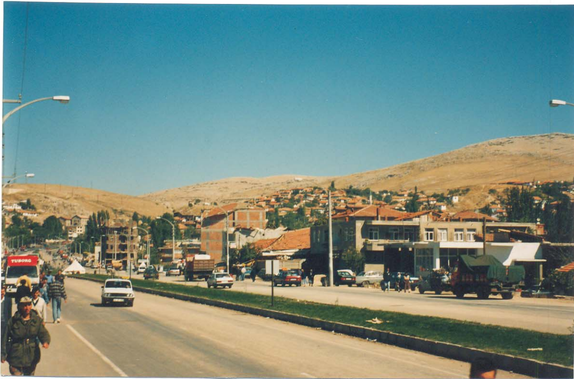
Fig. 3 View looking east at the part built on bedrock outcrops (limestone and marly limestone). At this particular section of the city, damage was limited.
