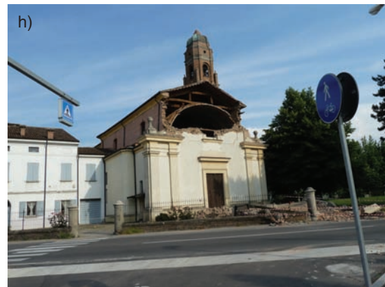
Fig. 33. The incurred damage of churches follows almost an identical pattern. The bell towers survived with only minor damage along the height. In most cases the top of the spire was damaged; a), b) church of San Marino at Buonacompria; c), d) church of San Francesco at Mirandola, very heavy damage. The bell tower collapsed after the second event; e) Santa Maria Maggiore, Cathedral of Mirandola; f) a view from the north towards S-E; g), h), two damaged churches in Mirandola.
