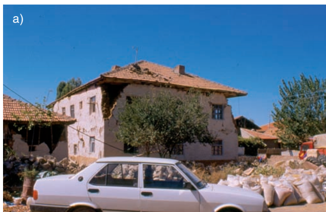
Figs. 35 a, b The damage to symmetrical masonry structures are symmetrical around the vertical vector. The well known diagonal cracks are not developed. The horizontal cracks at roof and first storey levels are due to vertical vibration of the roof and floor respectively. Typical is the detachment of all four top corners around the building. Dinar, Turkey, 1995 earthquake, /14/.
