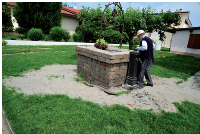
Fig. 12. Well with liquefied sand deposition due to violent ejection in San Carlo.
