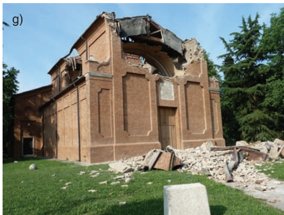
Fig. 33. The incurred damage of churches follows almost an identical pattern. The bell towers survived with only minor damage along the height. In most cases the top of the spire was damaged; a), b) church of San Marino at Buonacompria; c), d) church of San Francesco at Mirandola, very heavy damage. The bell tower collapsed after the second event; e) Santa Maria Maggiore, Cathedral of Mirandola; f) a view from the north towards S-E; g), h), two damaged churches in Mirandola.
