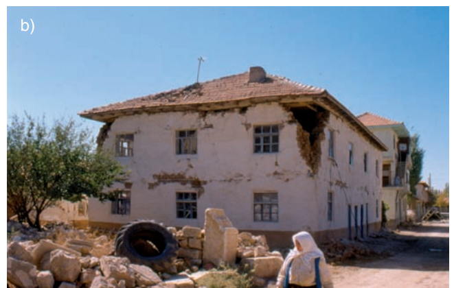
Figs. 35 a, b The damage to symmetrical masonry structures are symmetrical around the vertical vector. The well known diagonal cracks are not developed. The horizontal cracks at roof and first storey levels are due to vertical vibration of the roof and floor respectively. Typical is the detachment of all four top corners around the building. Dinar, Turkey, 1995 earthquake, /14/.
