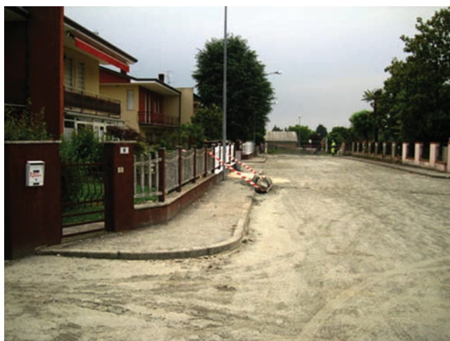
Fig. 15. San Carlo residential area. Big amounts of liquefied material have covered roads throughout the city.
