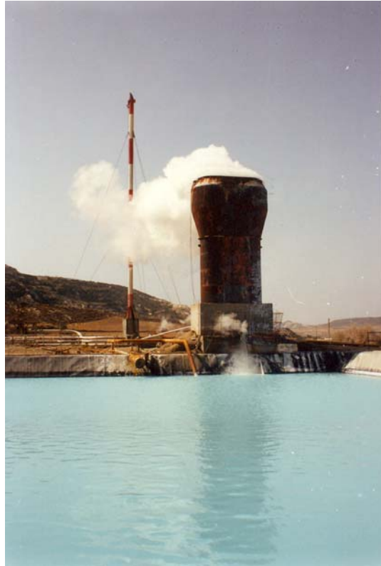
Figure 2. Toxic geothermal fluids in an open tank at Zefiria -Milos Island. The reservoir is water tight to avoid land contamination. Due to the limited volume available, fluids were inserted into deep geologic strata through an adjacent fault zone.
